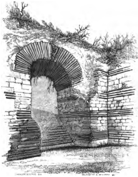
1. Roman Masonry and Arch formed of Roman bricks or tiles; from Porchester Castle, Hampshire.
